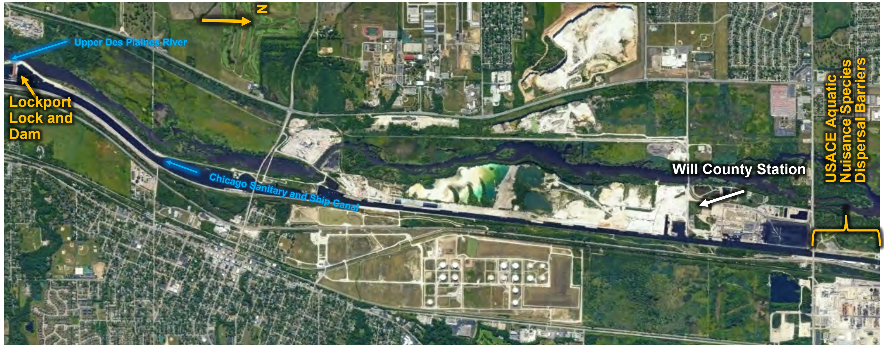
Location of the Will County Station Thermal Discharge into the Chicago Sanitary and Ship Canal of lower Lockport Pool.
